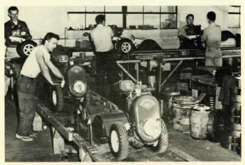
Improvements to the machine were accompanied by improvements in the manufacturing process. By the mid-fifties, the **ROTOTILLER** factory was capable of turning out a new tiller every 6<sup>1</sup>/<sub>2</sub> minutes. In the photo above, Joe Zakrzewski checks final assembly. Four members in two generations of the Zakrzewski family are still turning out Tillers in Troy.
